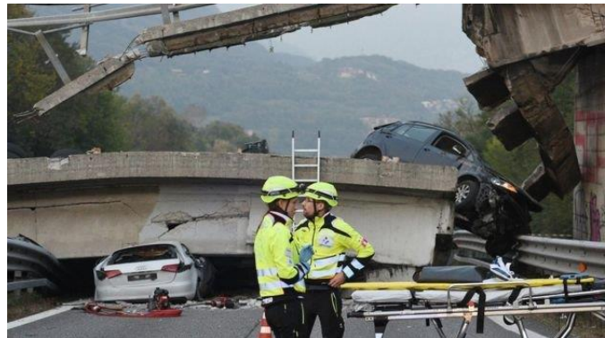
Collapse of a flyover causing casualties, 2016.
